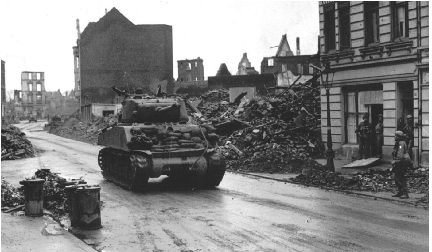
Some Shermans were fitted with a 76mm gun from February 1944 in time for the northwest Europe campaign.
